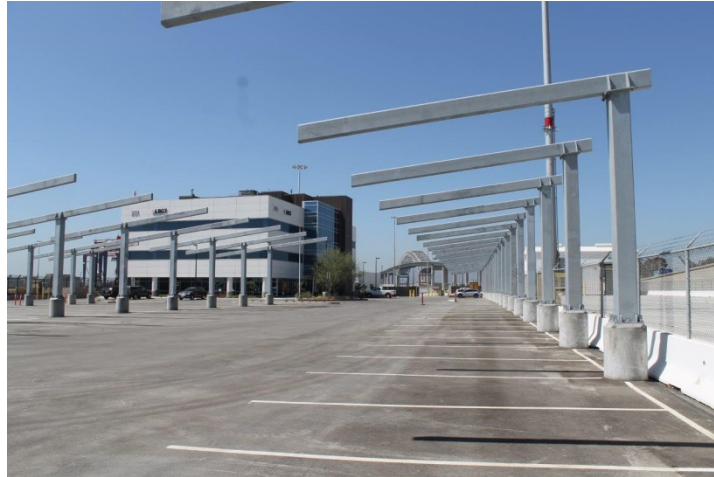
Cantilevered Gantry/Canopy Structure
