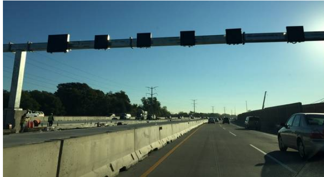
Overhead Gantry Structure
